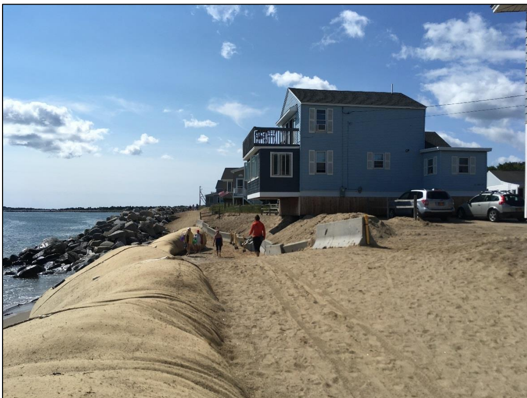
12. Geotube, rip-rap, and infrastructure at risk at Camp Ellis, Stop 5.
